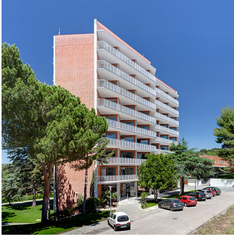
“Santo Tomás de Aquino, Aquinas” Residential College Colegio Mayor Santo Tomás de Aquino “Aquinas” Madrid. Specific Restoration, Preservation and Restructuring. Design, Construction Supervision and Technical Construction Supervision. BIM Project. 7.995 m 2 | 2010 - 2014
