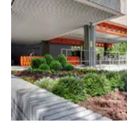
“Isabel de España” Residential College Colegio Mayor “Isabel de España” Madrid. Restoration, Renovation and Preservation project. Design, Construction Supervision and Technical Construction Supervision. 1.300 m 2 | 2012 - 2014
